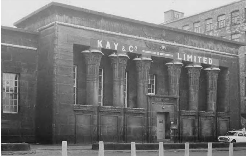
Plate 162 Temple Mills, Marshall Street, Leeds (1842), by Joseph Bonomi Jr and James Combe of Leeds. This was the most coherent attempt to adapt an Egyptian temple to a commercial building. John Marshall of Leeds, keen to advertise his new flax-spinning mill, commissioned David Roberts to make designs, and Roberts contacted Bonomi for help. The main influences are Edfu and Dendera, and the chimney was an obelisk. Even the machinery inside was in the Egyptian style, chosen no doubt because the Ancient Egyptians used flax for the production of linen. Photograph of 1979 (JSC).
